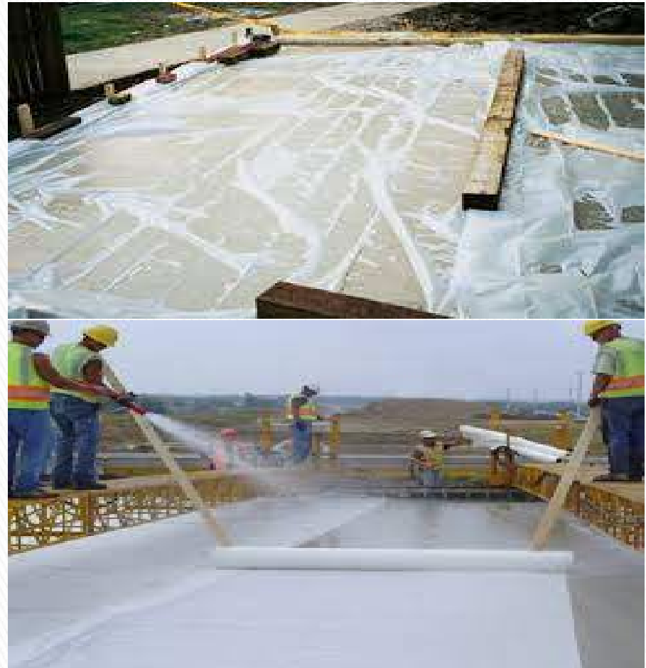
Curing of Cement Concrete
